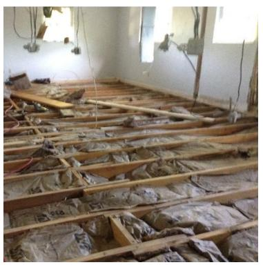
We replaced the sub floor on the second story to remedy an issue with termites, and we reconfigured some walls on both floors to open up the floor plan and relocate some of the bathrooms.
